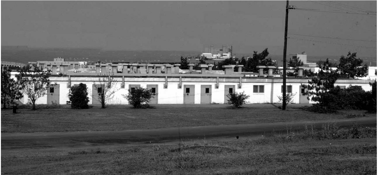
The Poultry Virus Isolation building situated to the west of the veterinary college on the campus
