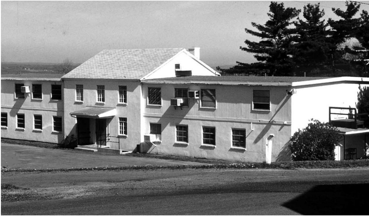
The Levine Laboratory after the wings were added to and after a second story was constructed over both wings in the mid 1960s
