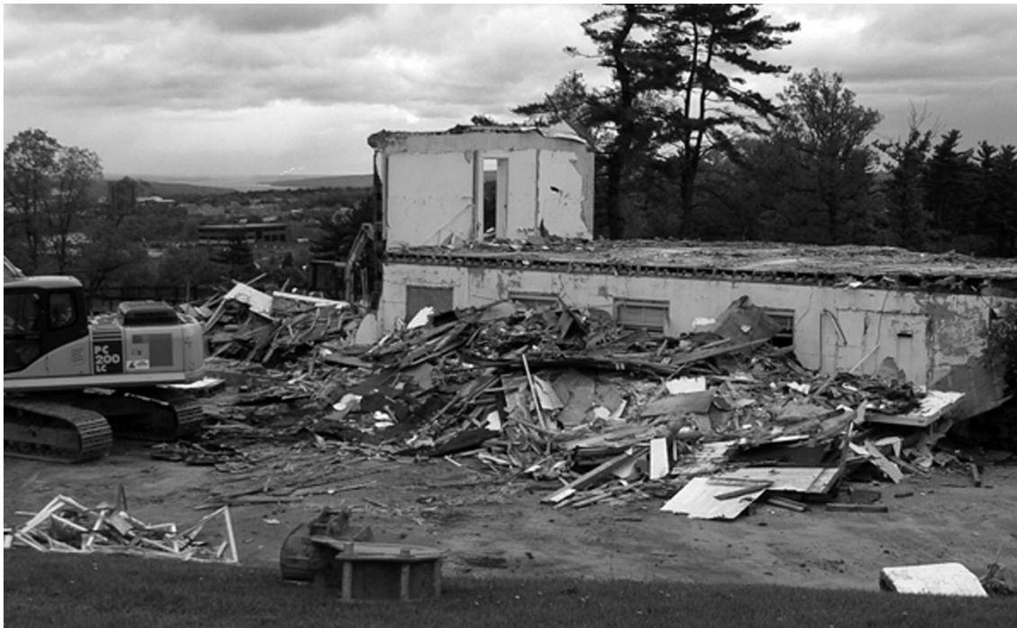
Demolition of the Levine Laboratory - May 2008
